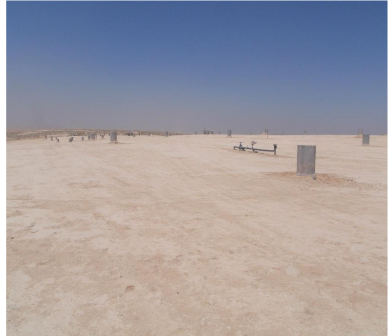
Landfill cover and gas wellheads protected by concrete rings
